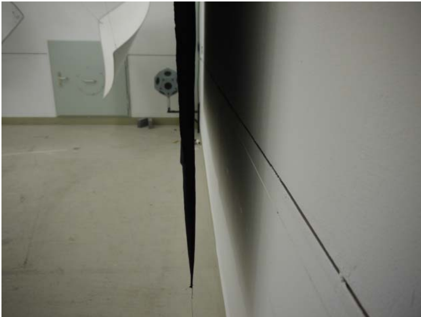
Figure B2. Distance of 200 mm between fabric and wall; without enclosing frame
